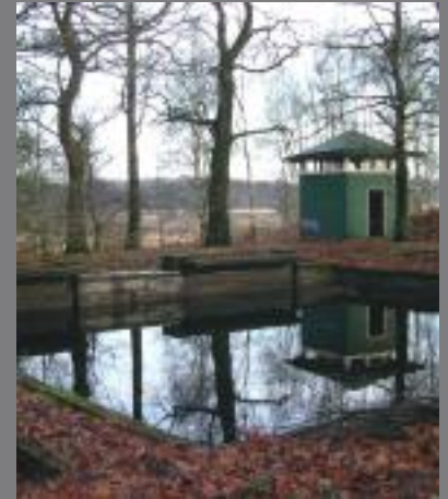
In the summer, building E's cooling pool was cleaned by the village inhabitants and provided with fresh water so serve as a swimming pool. The antenna coupling house was then used as a pool house
